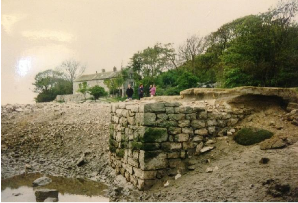
Plate 22. The southern end of Site 2D being eroded from the saltmarsh. Photo by Barry Ayres dated c.1995. Note at least seven courses exposed in this image.
