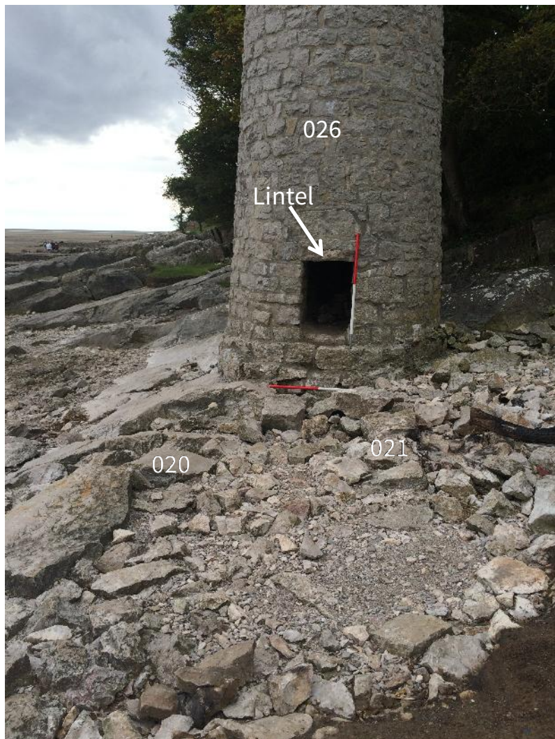
Plate 34. Lower elevation of Chimney 026 showing the east-facing opening and foundations 021/021
