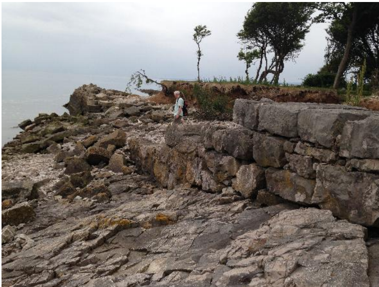
Plate 2. Substantial L-shaped ?revetment wall
