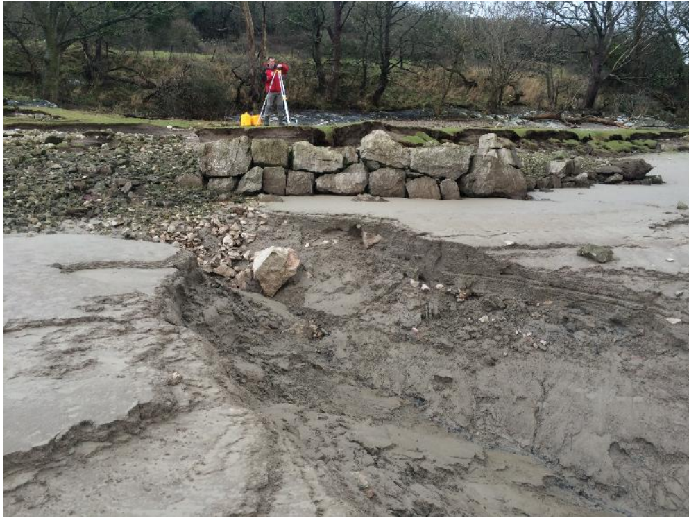
Plate 45. Wall 017 showing the deep channel that had opened up in front of the structure during the winter of 2015/6. February 2016
