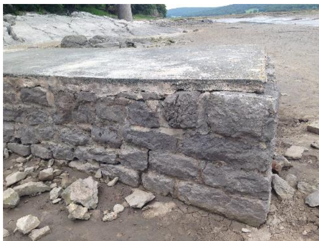
Plate 7. Jetty situated to the south-west of the Chimney
