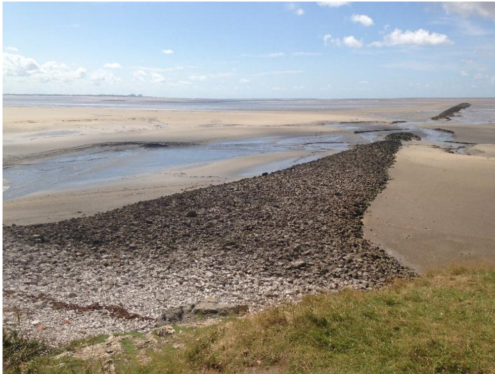
Plate 4. The remains of the embankment in 2015 formed of stone cobbles extending out into Morecambe Bay from Jenny Brown's Point, looking south-west
