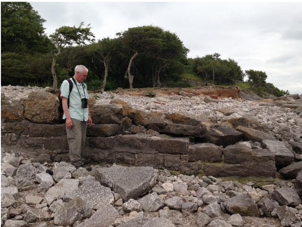
Plate 11. Volunteer Simon Williams inspecting the north east-south west wall forming the southern side of the quay. The rubble of the embankment is in front. (August 2014)
