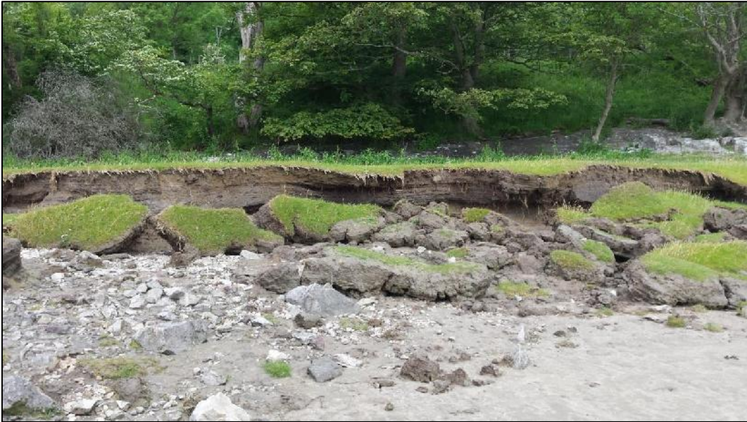
Figure 9: Erosion of the salt marsh edge. View to the north.
