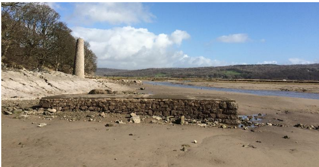
Plate 46. Western elevation of possible jetty/quay ( 100/101 ) with the chimney ( 026 ) in the background, looking east. March 2015
