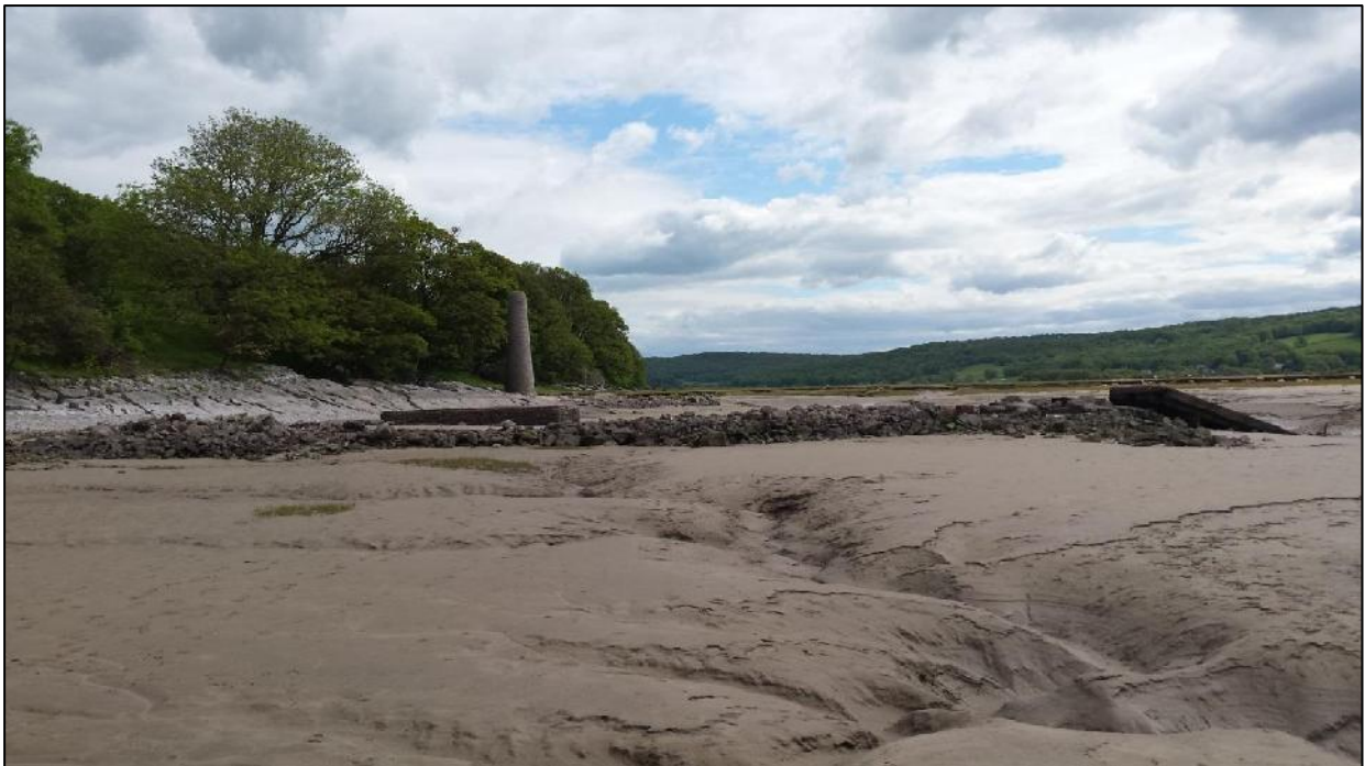
Figure 8: The foreshore at Jenny Brown's Point, showing the collapsed bridge (foreground), the small stone quay (PRN 520; middle ground) and chimney (UID 181949/PRN 4821; background). View to the northeast.
