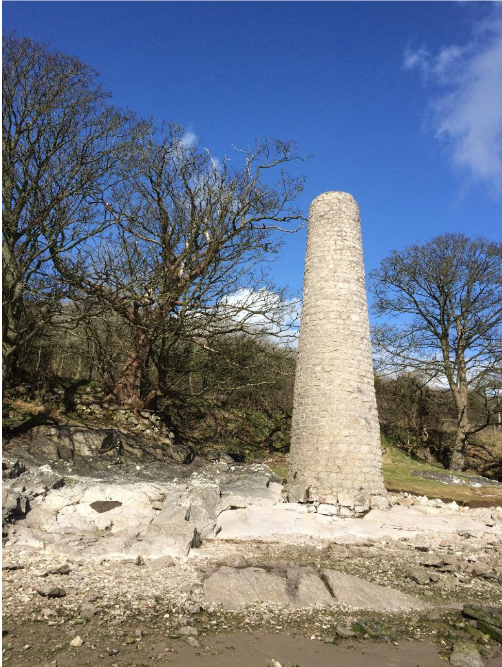
Plate 13. The chimney at Jenny Brown's Point (Site 2A), looking east (March 2015)
