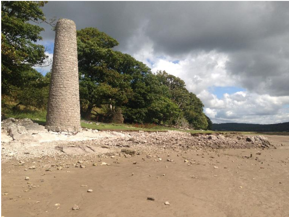
Plate 14. The chimney site (Site 2A) to the left with the remains of the revetment/quay (Site 2C) to the right, looking north-east (August 2014)
