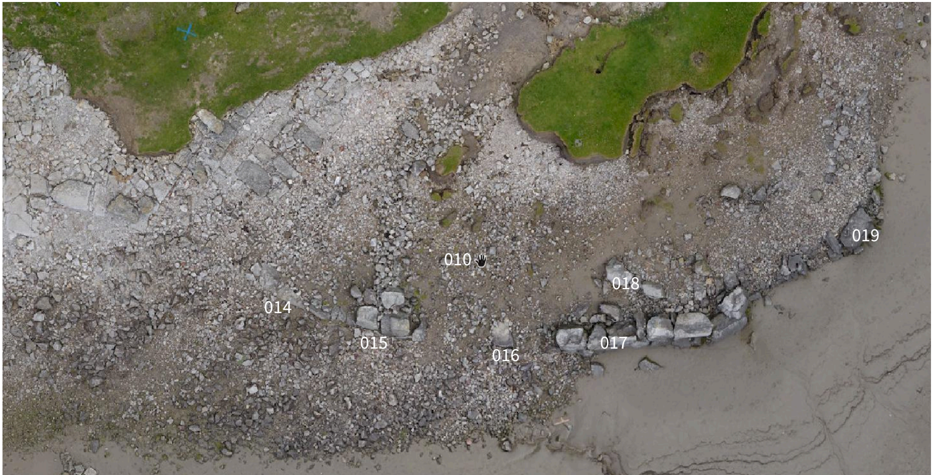
Plate 42 Aerial plan view showing the possible revetments walls 014-019
