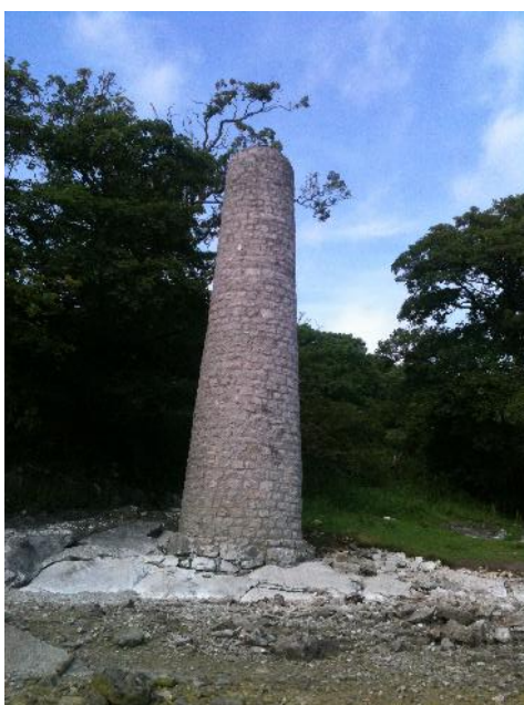
Plate 4. Chimney at Site 2
