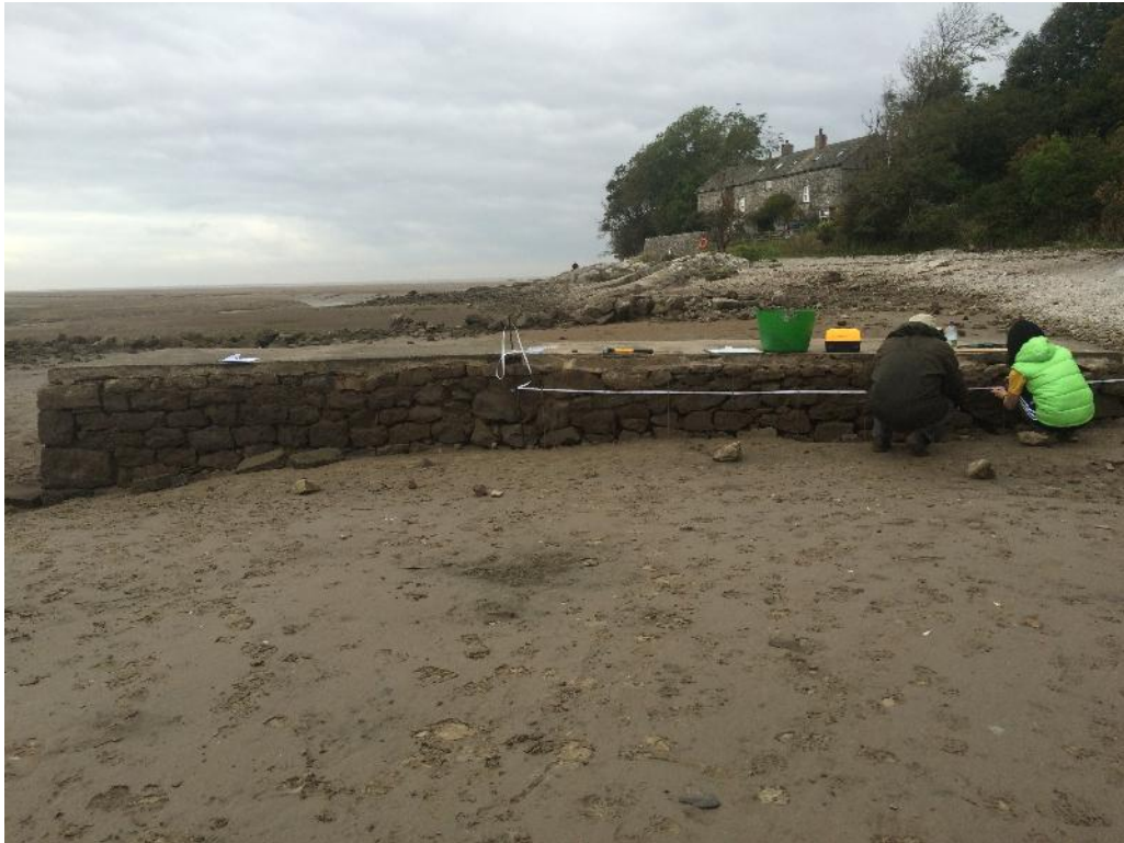
Plate 49. Volunteers recording the eastern elevation of the possible jetty/quay (100/101) during August 2015
