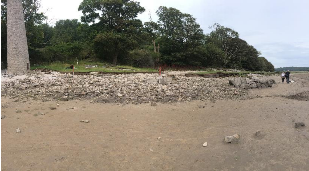
Plate 43. Ranging poles define the north-western end of (014) left, wall (015) (centre) with wall (017) to the right, August 2015
