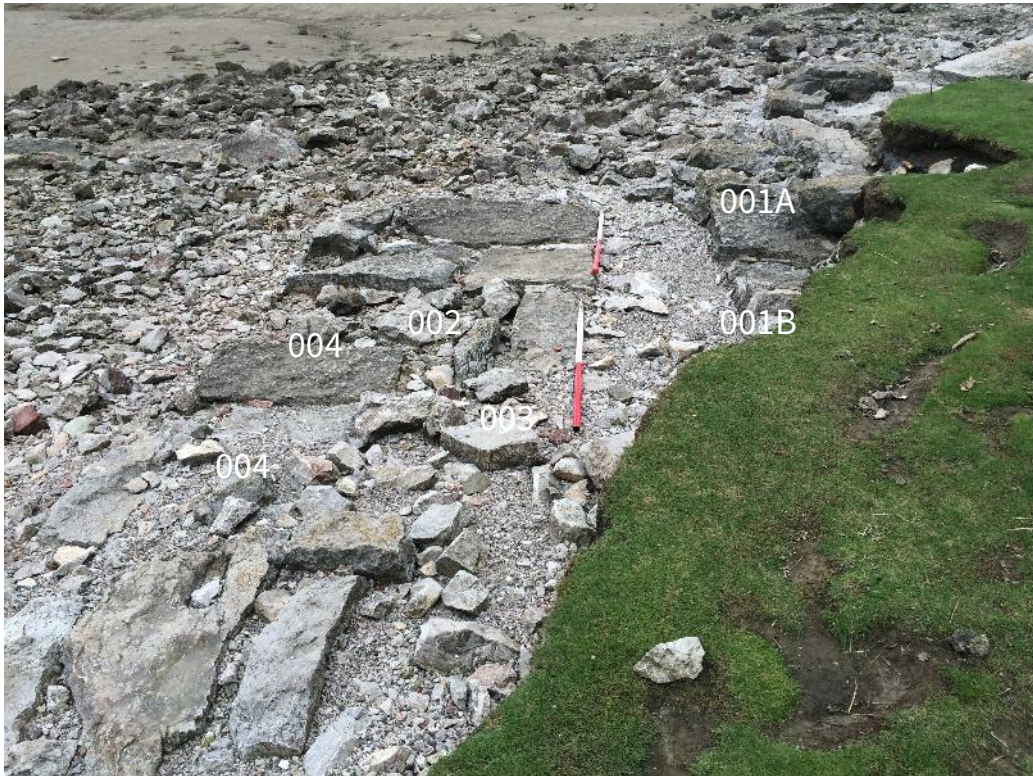
Plate 37 North-east to south-west aligned wall foundations, noted to the south-east of the chimney, looking south-west
