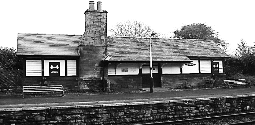
Figure 1: The waiting room at Silverdale Railway Station
